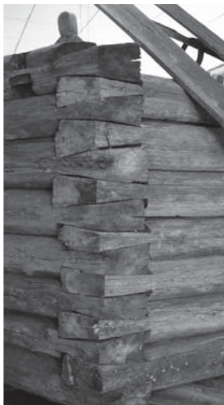
The corner of a reconstructed timber fortified wall of the type used by both Volga Bulgars and Russians. The joints are cut in such a way that the logs cannot be pulled outwards. (Photo V. Shpakovsky)
